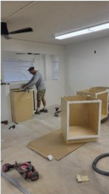
Installation of front counter cabinets.
