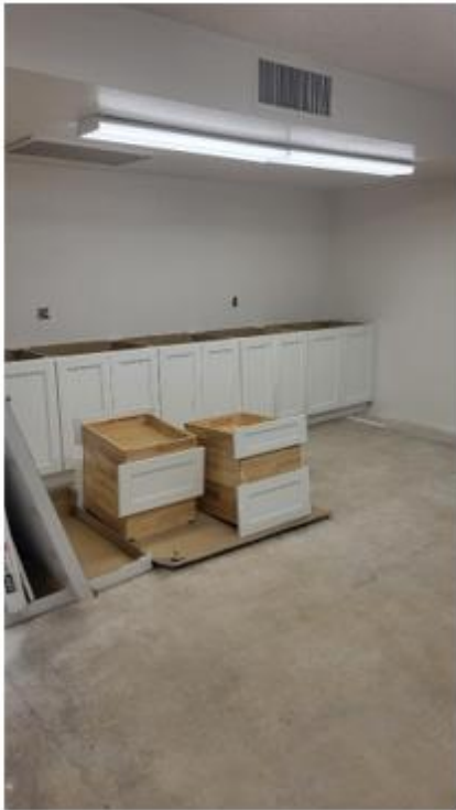
Cabinets installation for back Counter.
