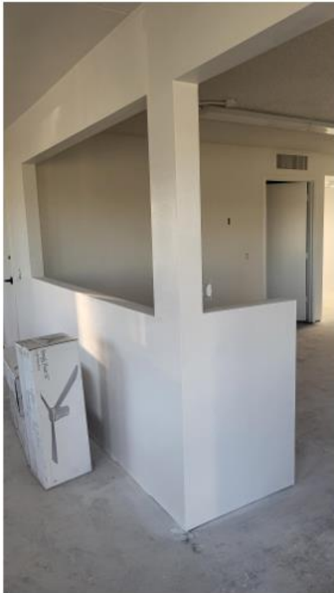
Front Counter has been reconstructed Drywalled and painted.
